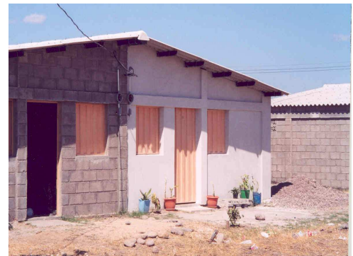
Low-cost shelters in Honduras built with a Matching Grant.
